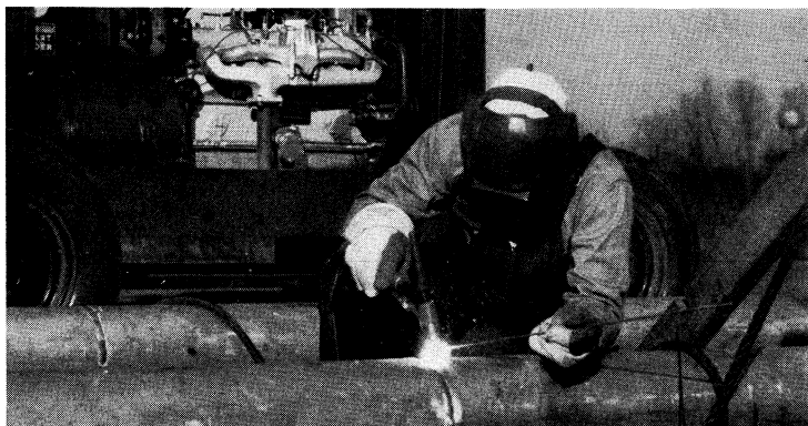
Tungsten arc welding of an aluminum pipe line
