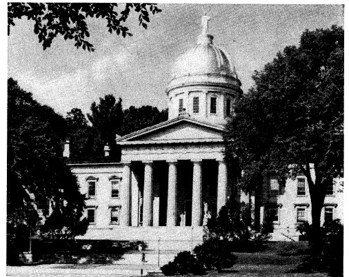
Vermont state house at Montpelier. Constructed of native granite, the capitol was first built in 1836, renovated in 1859. The portico is designed after the Greek temple of Theseus, Athens
